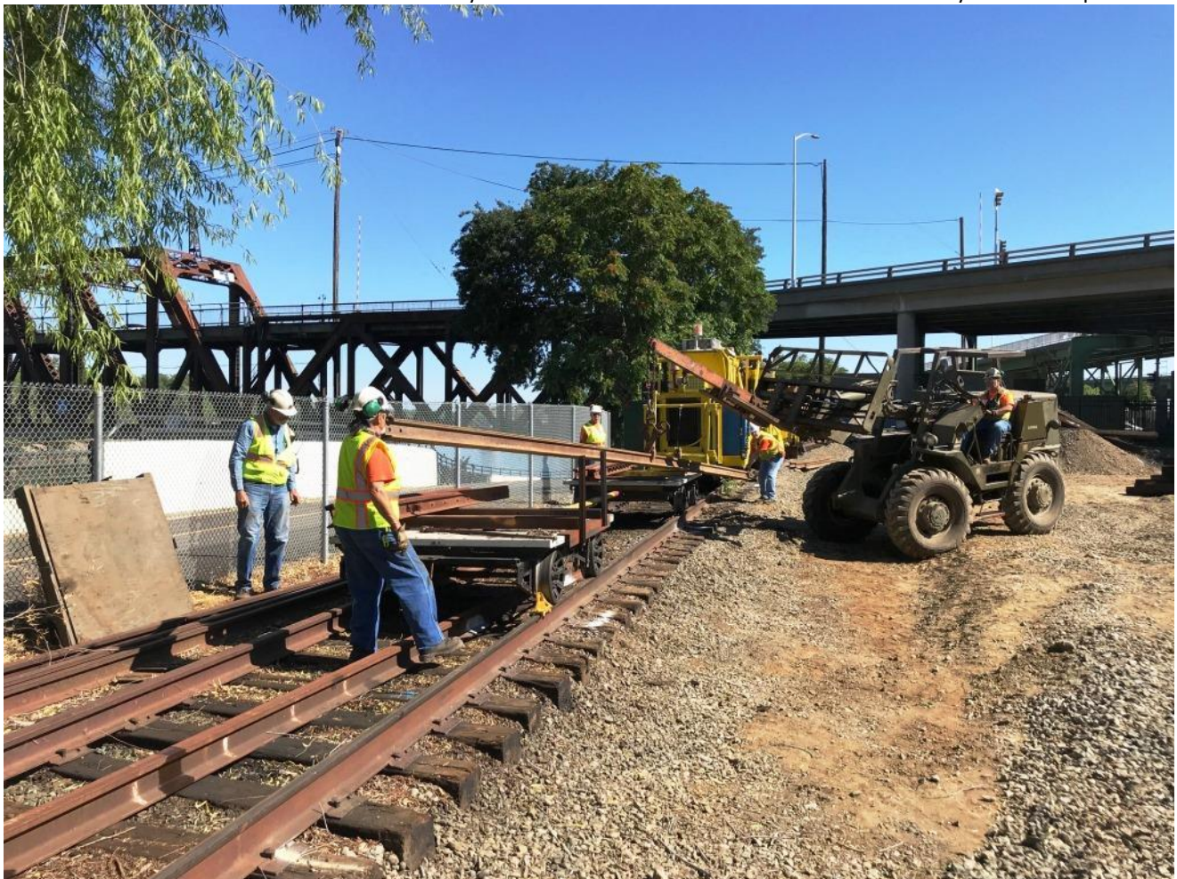
Ed and Bill guide the removal of the rail by Mike F. on GM2
