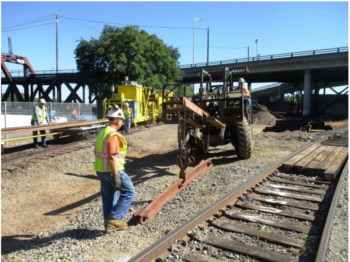
Clem works with Mike F. on GM2 as one of the guard-rails is moved aside
