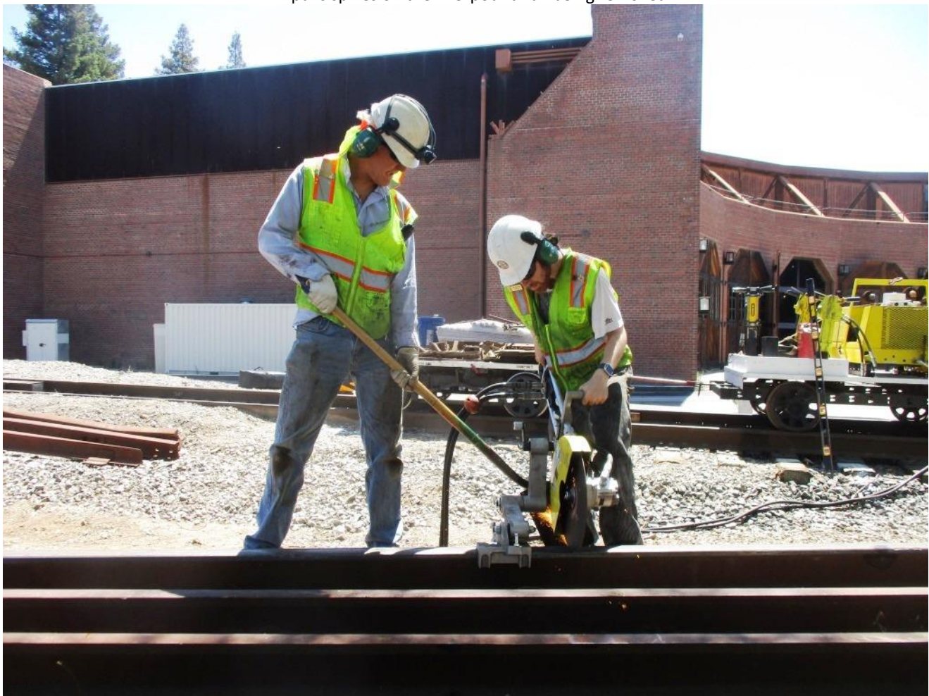
Steve uses a shovel as a spark-arrestor as Matt slices through the rail with the hydraulic rail-saw
