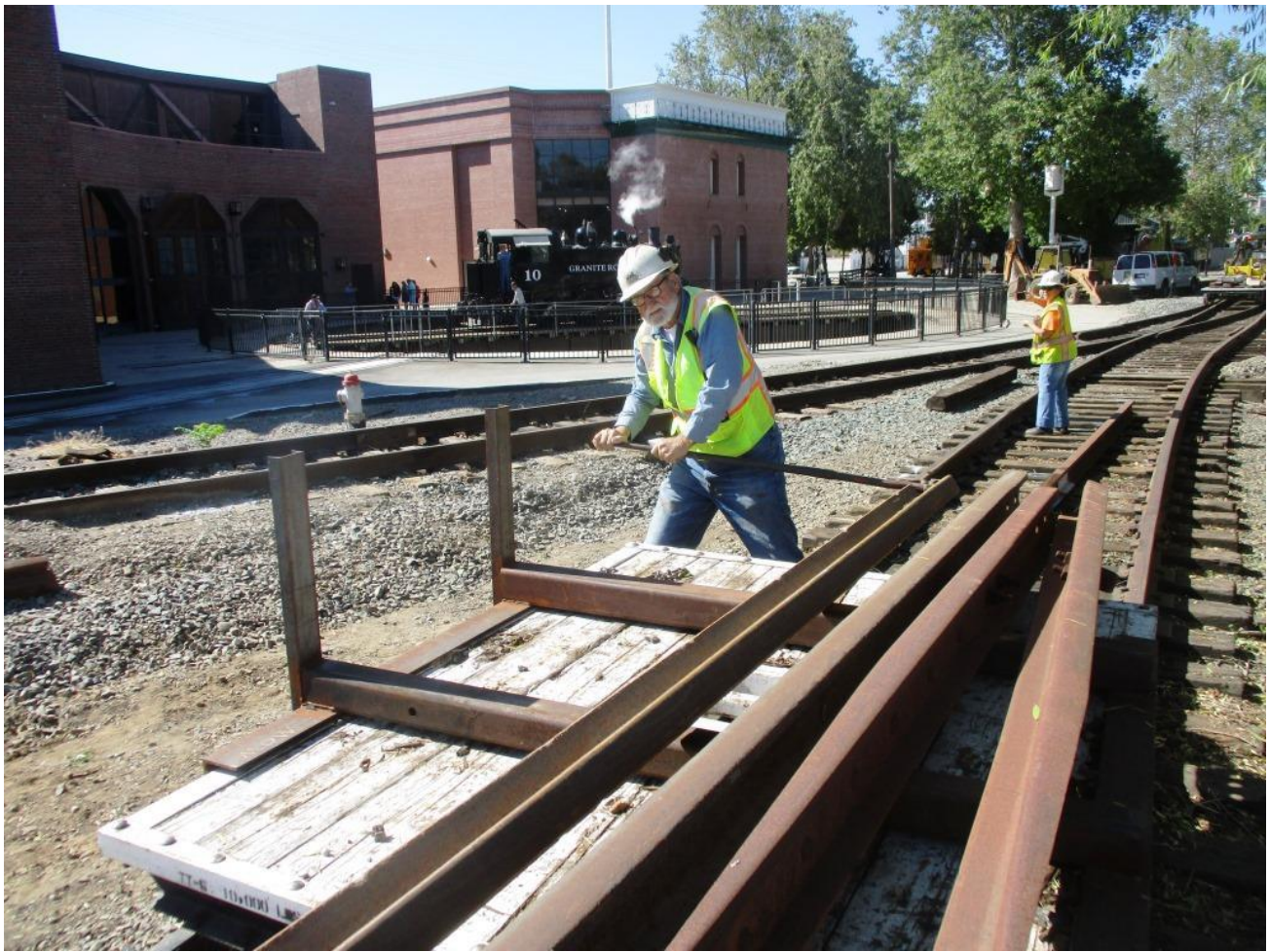
Alan uses a rail-fork to turn a rail upright
