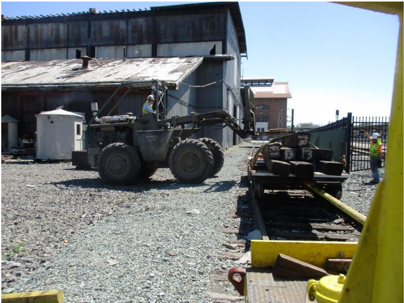
Next, Joe guides Steve on Big Green in the placement of a pallet full of switch-tie plates
