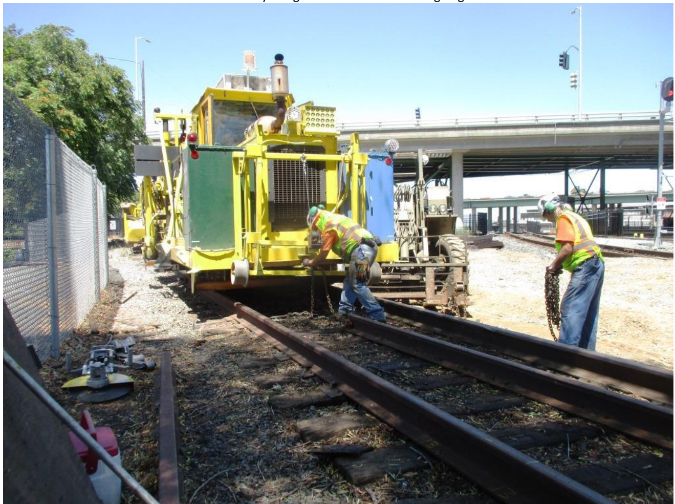
Because GM2 is in the way and out of commission, the Team invokes Matt's plan to use the tamper to pull the next rail into position
