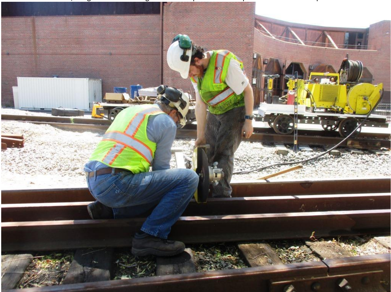
Alan and Matt set up the hydraulic rail-saw
