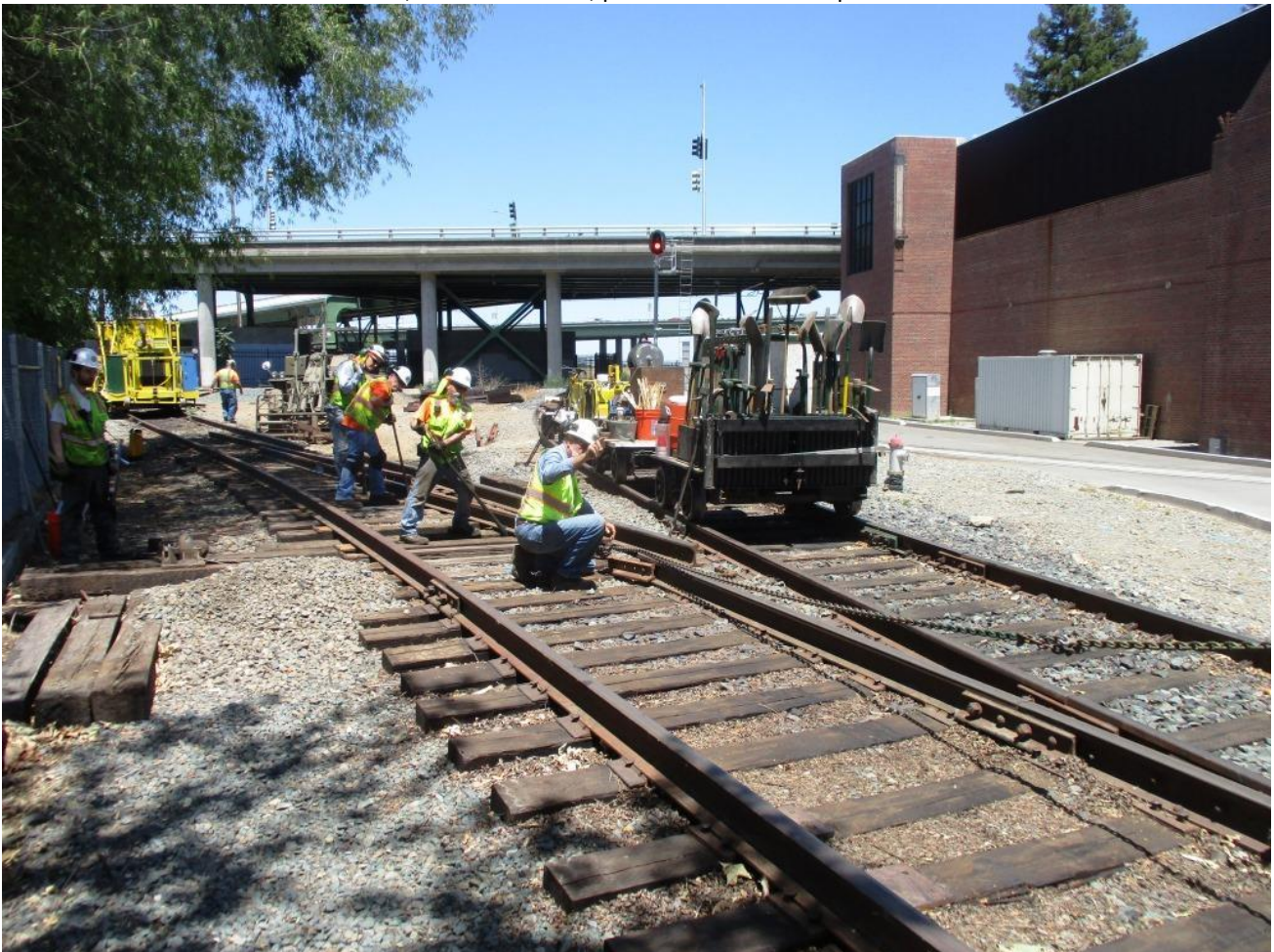
Alan directs Ed on the back-hoe as Joe, Bill, and Steve use lining bars to guide the rail to its final resting place
