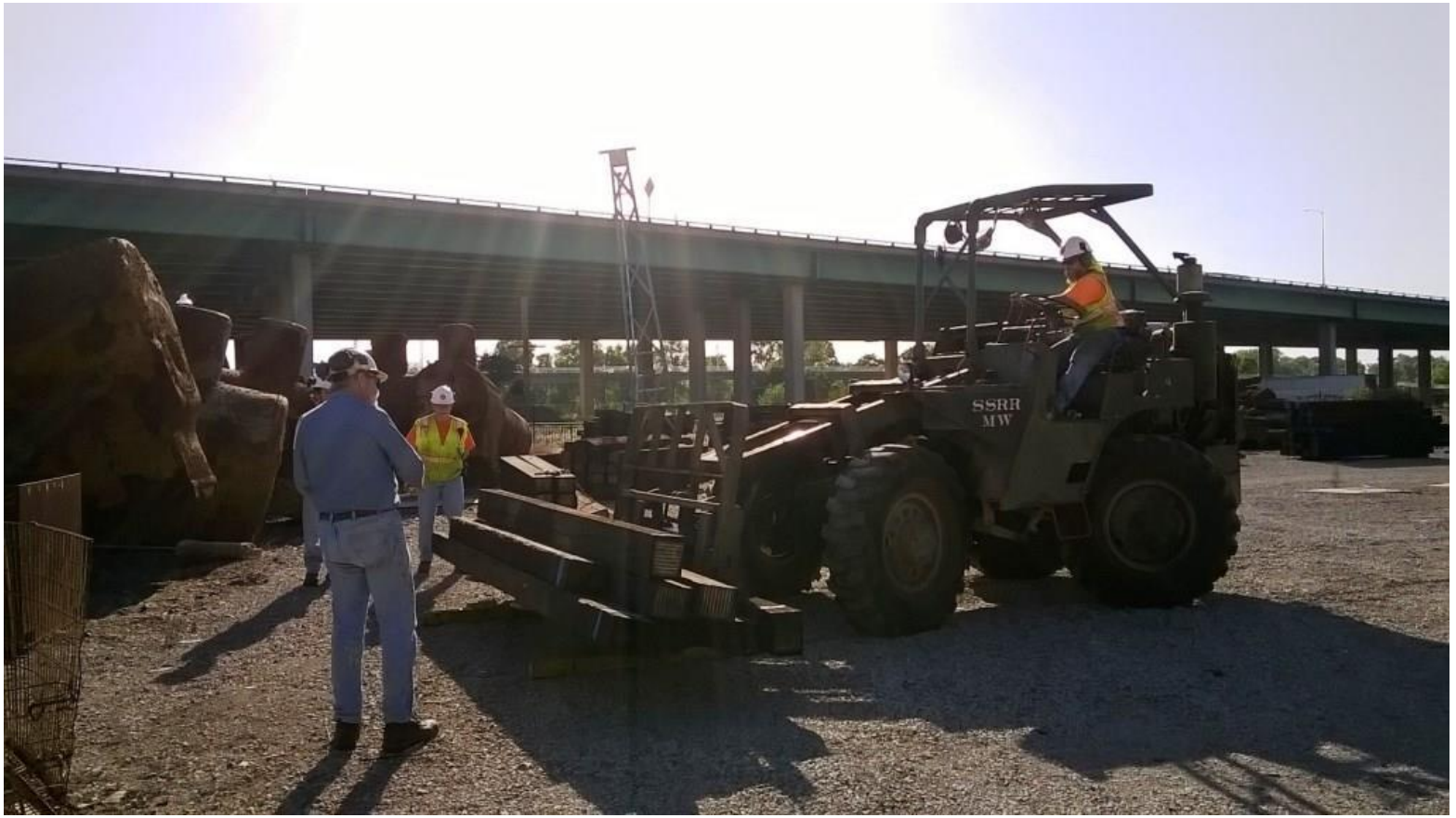
Joe, on Big Green, grabs the pile of extra-long switch-ties
