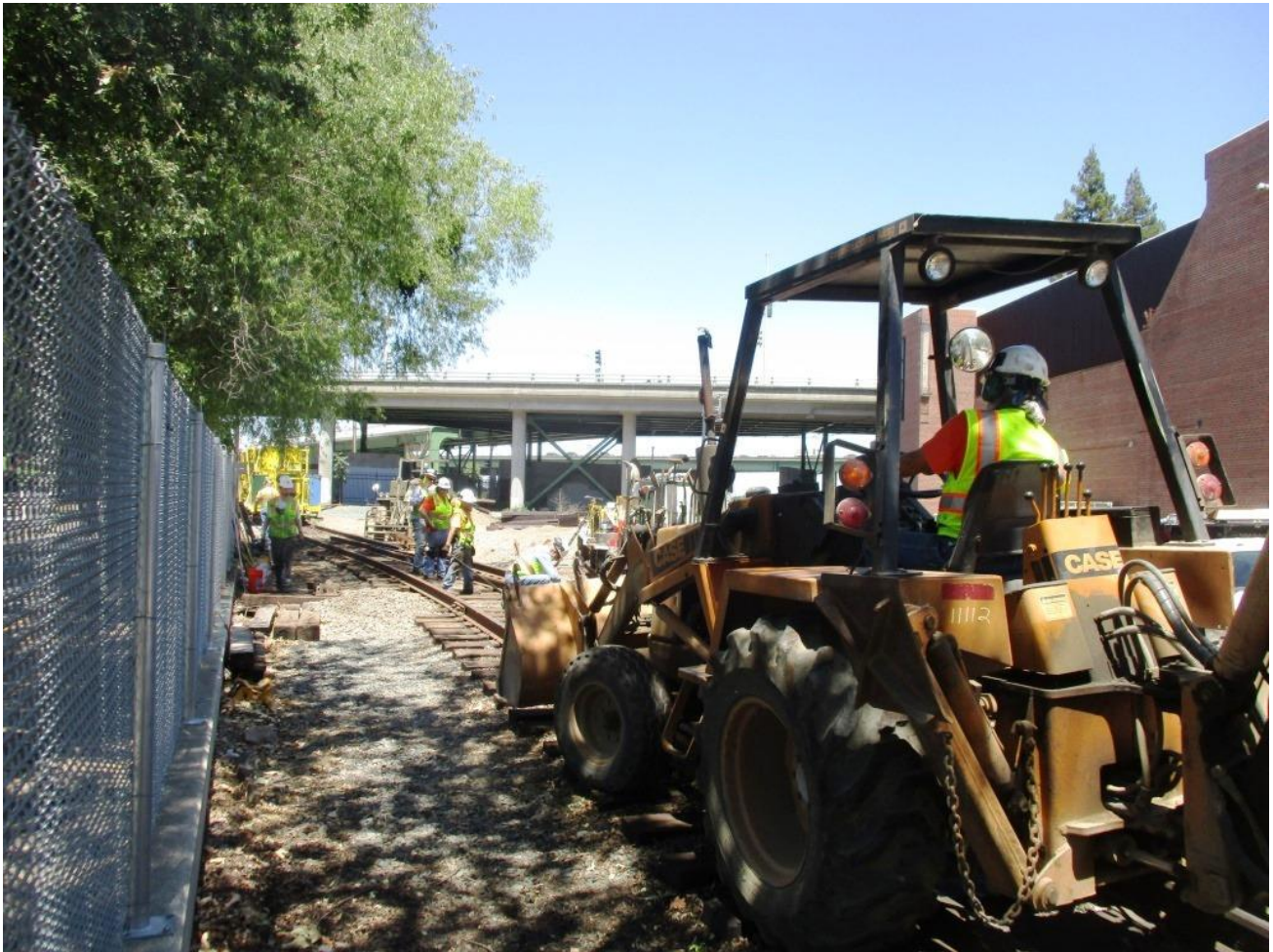
Ed, on the back-hoe, pulls the new rail into place
