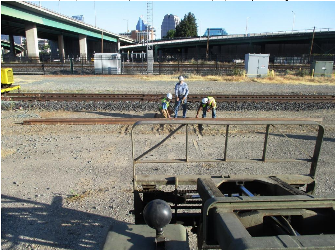
Second try: Kyle, Alan, and Dave indicate the balance point for where the Big Green Machine should pick up the rails
