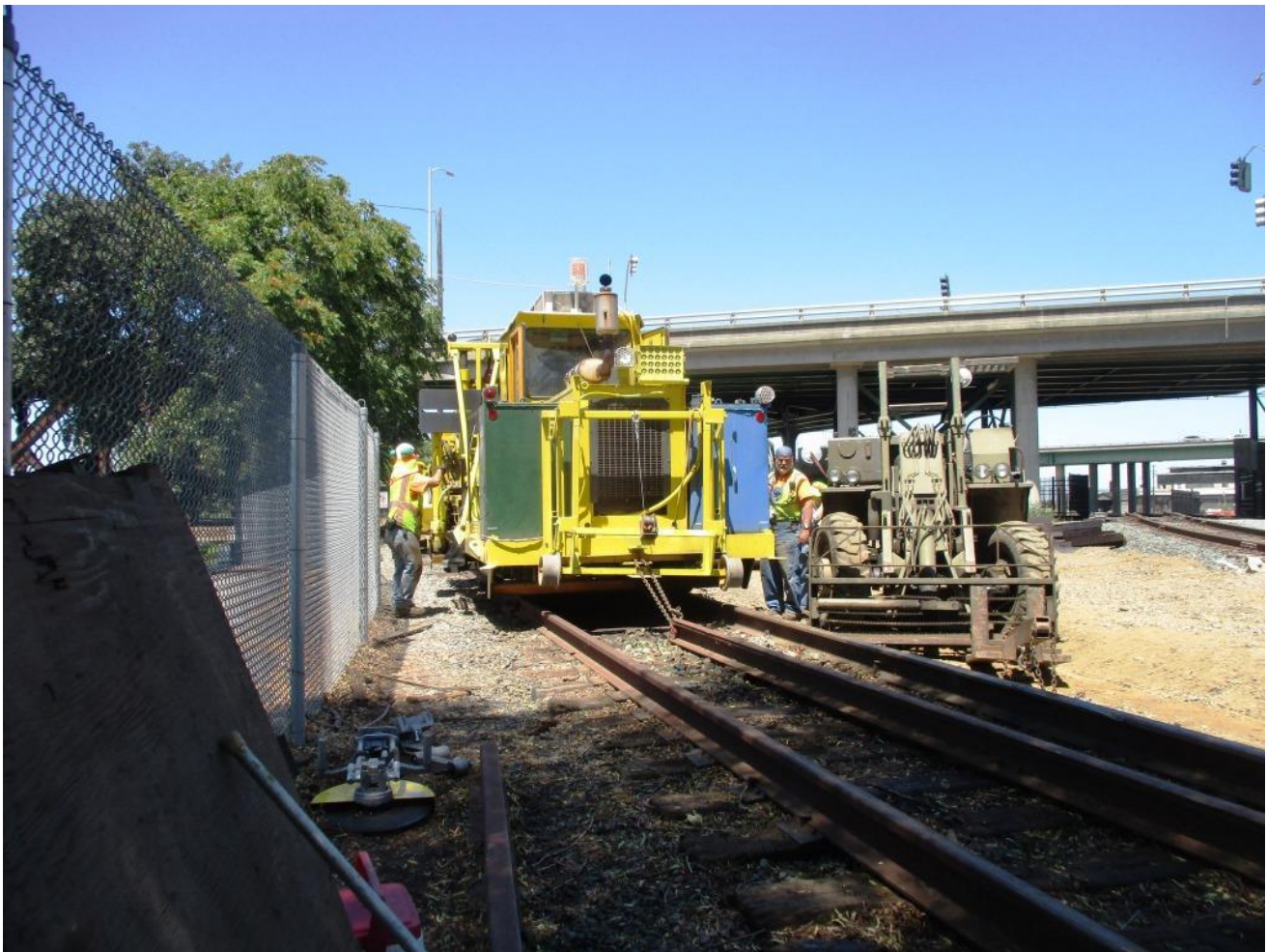
Joe guides Matt in the tamper from the ground as it pulls the rail up the line
