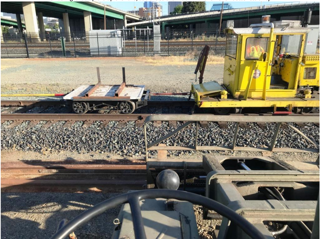
With the rails balanced on the forks, Chris brings in the Kalamazoo and flatcars for loading
