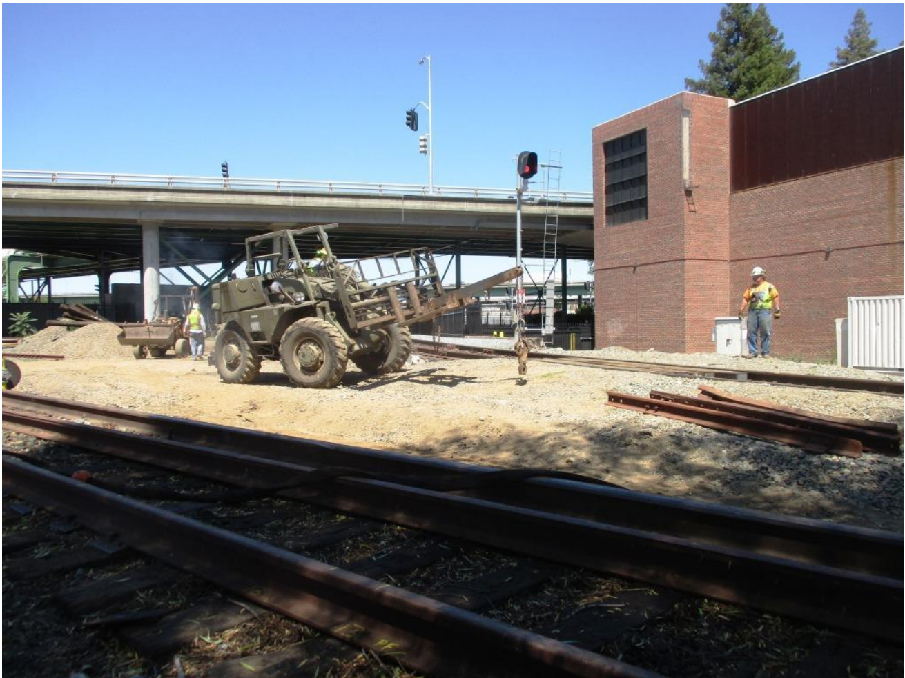
After being pulled out of the hole by the back-hoe, Heather on GM2 slowly coaxes it off the hill. Believe me folks, this was a major undertaking
