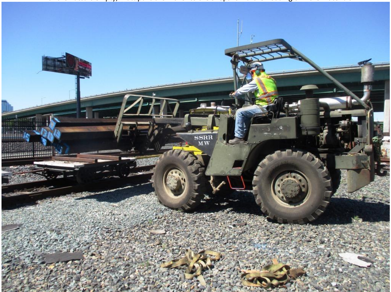
Over at the Shops, Steve on Big Green loads the extra-long ties onto the flatcar
