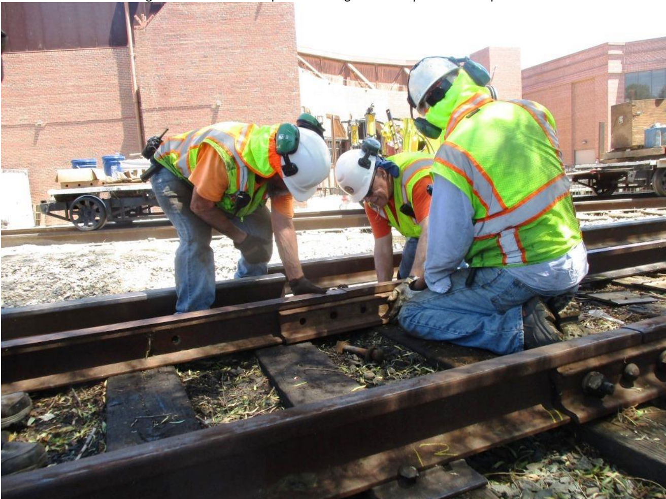
With everything where it's supposed to be, Joe, Bill, and Steve bolt the two new rails together
