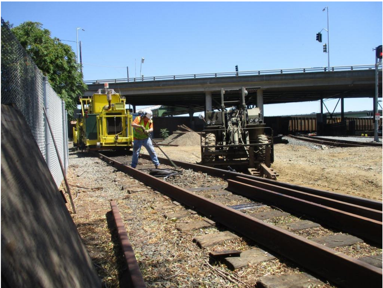
Bill pulls spikes on the 113-pound rail being removed
