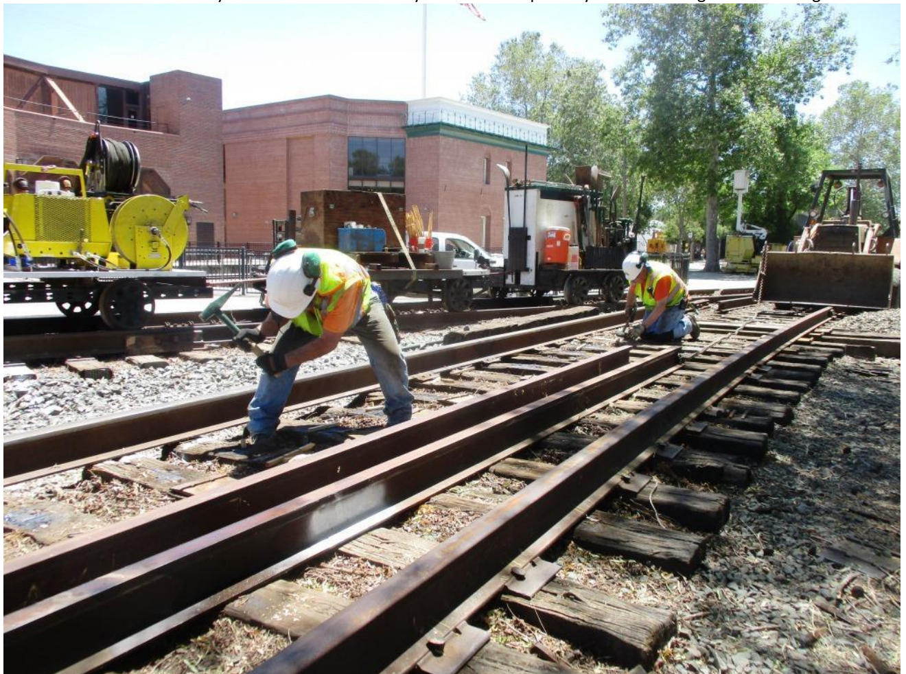
A chain is hooked between the rail to be moved and the back-hoe as Joe and Bill use tie-plugs to plug the old spike holes in the ties
